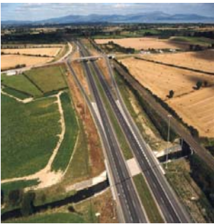
River Glyde Bridge
