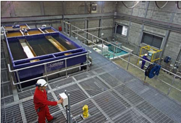
Effluent Treatment and Clarifier Area
